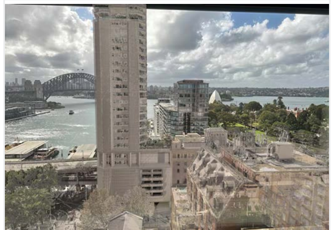
Point Cloud render of local site montaged
